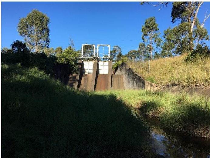
Figure 3-1 Original Grahamstown Dam spillway gates
