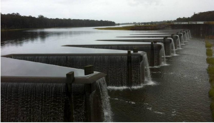
Figure 3-2 New Grahamstown Dam labyrinth spillway (source: Port Stephens Examiner, 2008)
